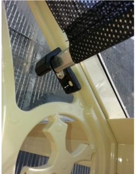
Left: To attach the hooks on a standard glazing bar, simply remove the nut from the spandrel and attach the hook with the same nut.
