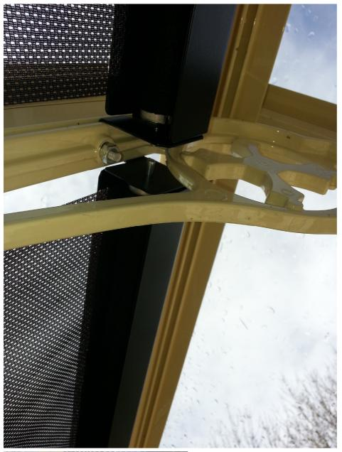
The best way to attach the blinds at the top of the roof is to clamp the tabs in between the spandrel and the glazing bar. Or when you have an A-frame, you can clamp the tabs in between the glazing bar and the A-frame channel in a similar way.
