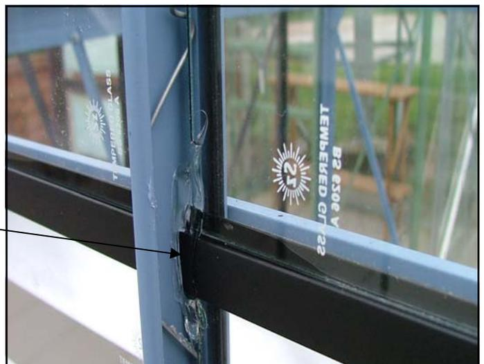
When inside your greenhouse you may notice a tiny shaft of light where the gutters (if applicable) and the ridge meet the gable end/s. This gap can also be filled with transparent silicone to avoid any leaking in these areas. It is also a good idea to silicone the corners of your base (if applicable) for the same reason.
