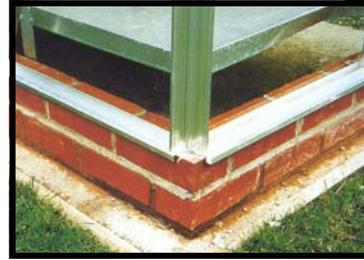
OVERLAPPING CILLS DEMONSTRATES THE NEED FOR ACCURACY WHEN BUILDING BRICK BASES.
