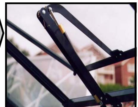
Fit the autovent so that it follows the **camber** of the roof.
